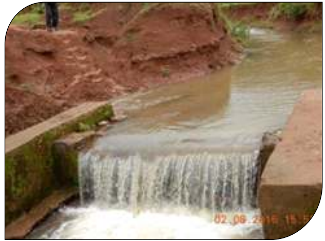
Check Dam at Gudiambaguda
