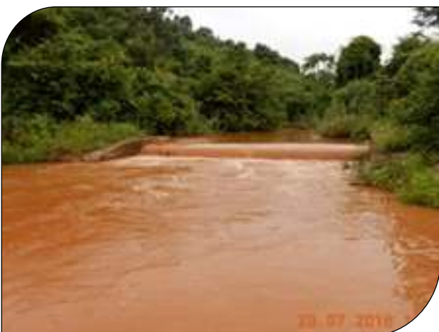
Check Dam at Totavalsa
