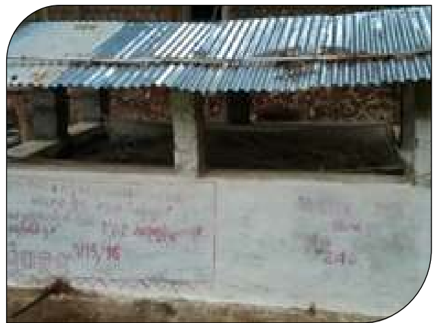
The vermicomposting pit in Chorimaliput
